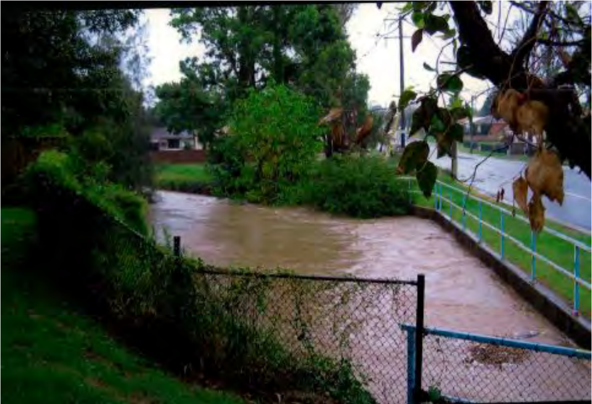
Upstream of Victoria Street culvert (date not nominated)
