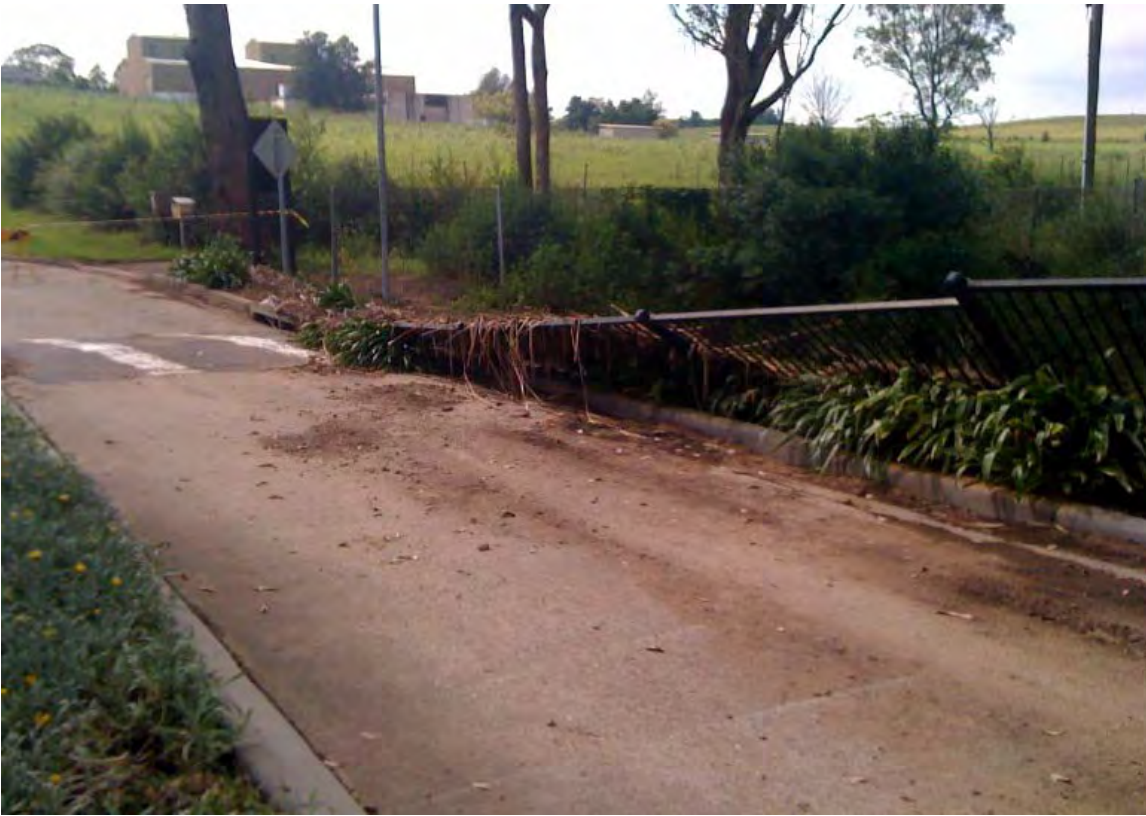
Fence at O'Connell St entrance to Western Sydney University
