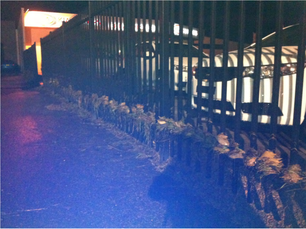
Debris mark approximately 0.2 metres above ground level at Morley Ave, Kingswood
