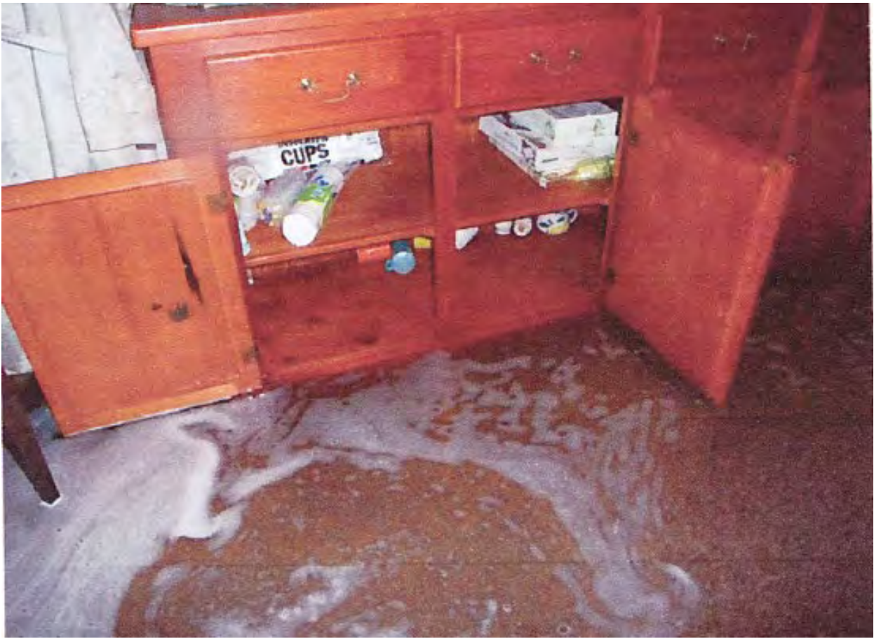
Above floor inundation at Stafford Crescent
