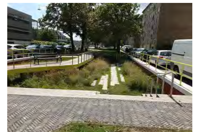
Fig. 73: Raingardens - a WSUD feature along streets in Chippendale, NSW
