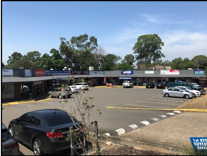
Poor presentation of shops in Mulgoa detracts from heritage character
