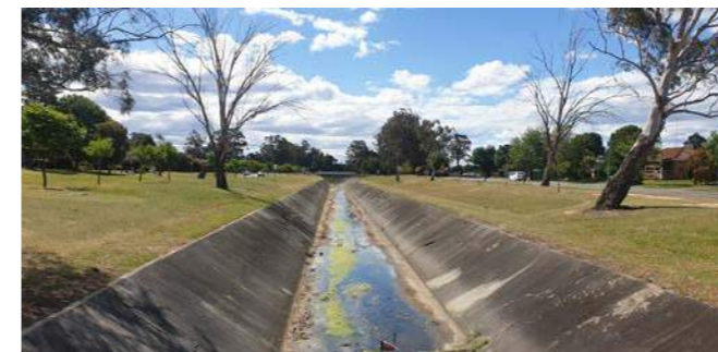
Figure 65. Existing View - Looking north towards existing pedestrian bridge
